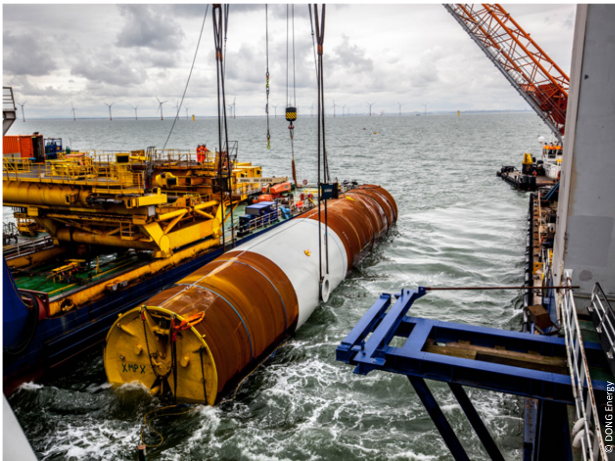
Monopile foundation installation
